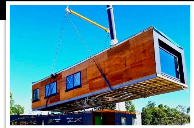
PREFABRICATED PRE-FINISHED VOLUMETRIC CONSTRUCTION
